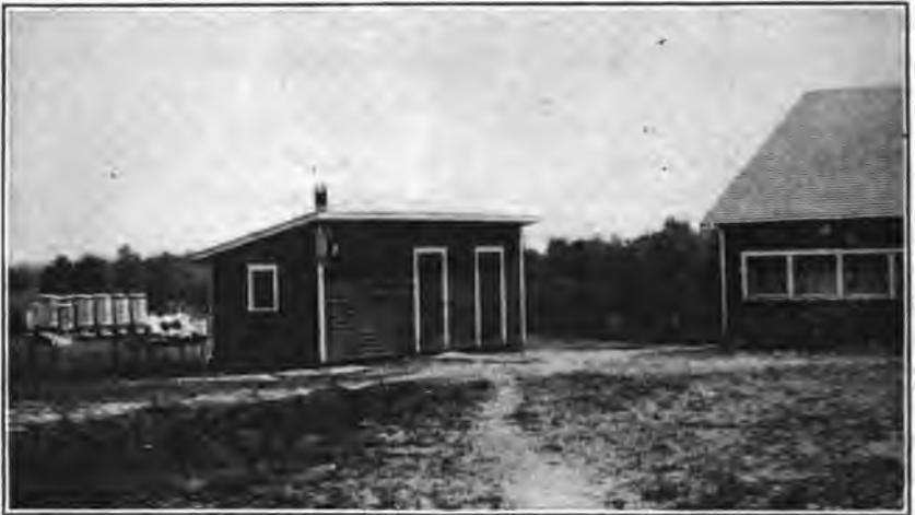
FIG. 4.—A sanitary but convenient and inexpensive milk house built according to plans recommended by the U. S. Department of Agriculture.
